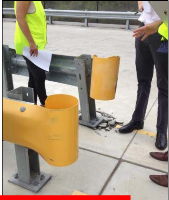
Minor impacts causing rigid post anchor failure
