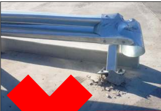
Minor impacts causing rigid post anchor failure
